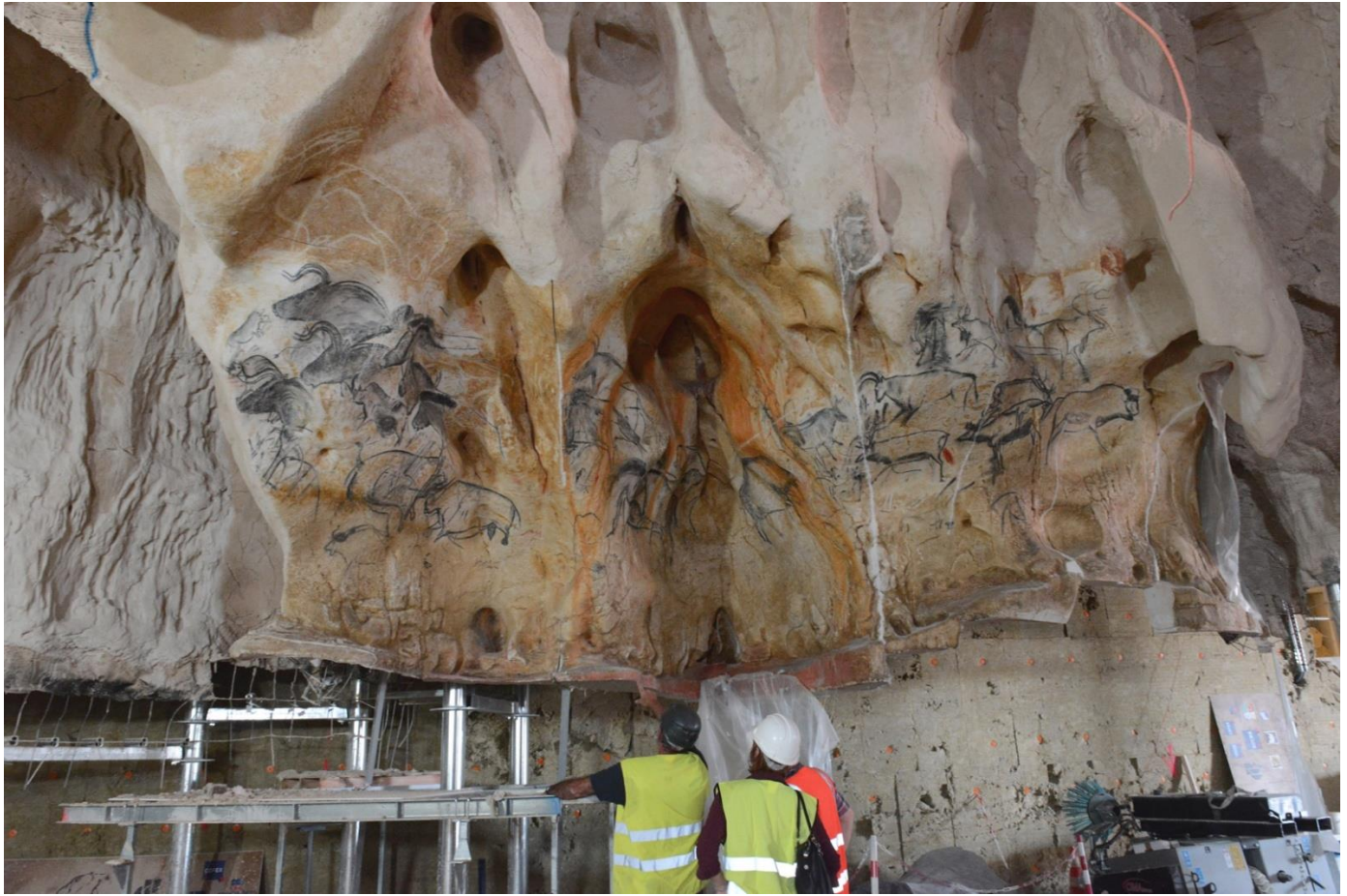
Figure 3. Insertion of the decorated panels on the Chauvet 2 replica construction site (photo C. Fritz)
